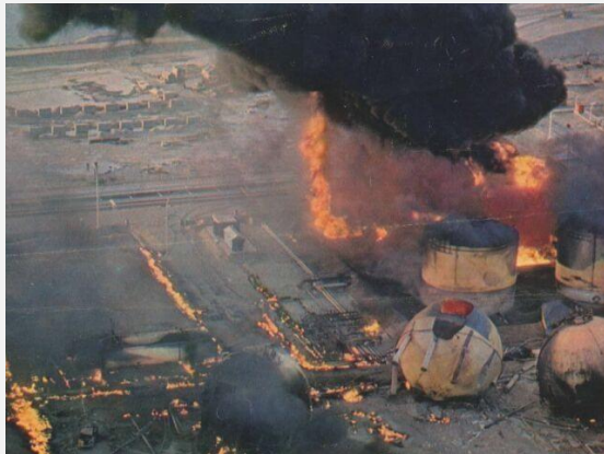
1966 : Feyzin oil refinery
